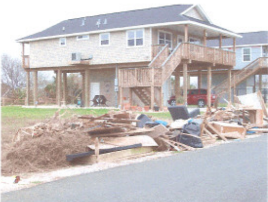
Just one of the many piles of debris on the street ready for pick up.
